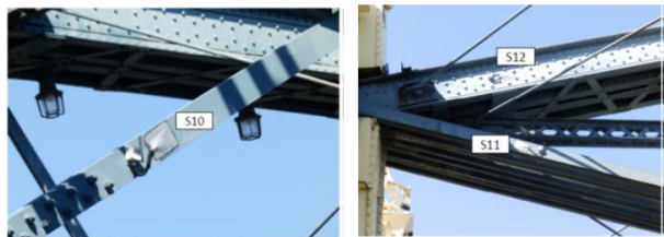
Wireless discrete sensors on the Smithfield Street Bridge , Pittsburgh. Photo credits: P. Rizzo
